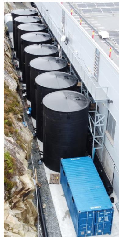
8 pcs. Ø3,8m & H6,3m filters (2000 kg feed per day)
